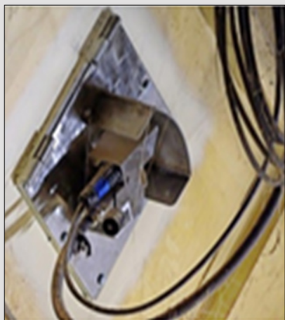
Figure 2. On-line NIR sensor installed in feed process (Courtesy of Dumoulin, Belgium. Projet FIRST Dumoulin-CRA-W).
